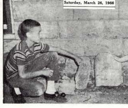
Mrs. Thomas and Johnny examined "flying saucer damage." Concrete reinforcement sheeting was broken, sand swirled.
